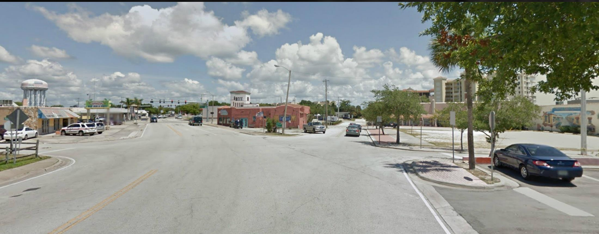
Florida Avenue – “Before”
